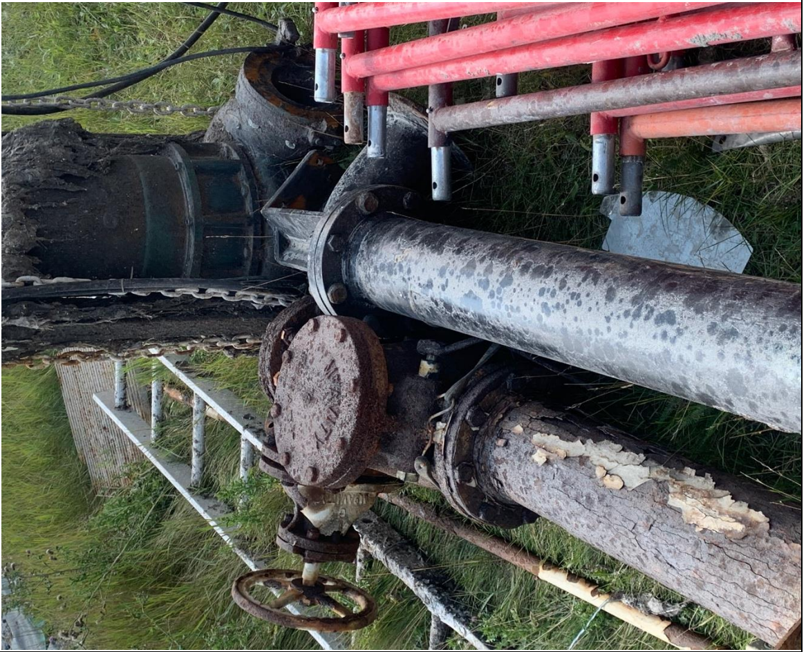
Lift pumps in poor condition
